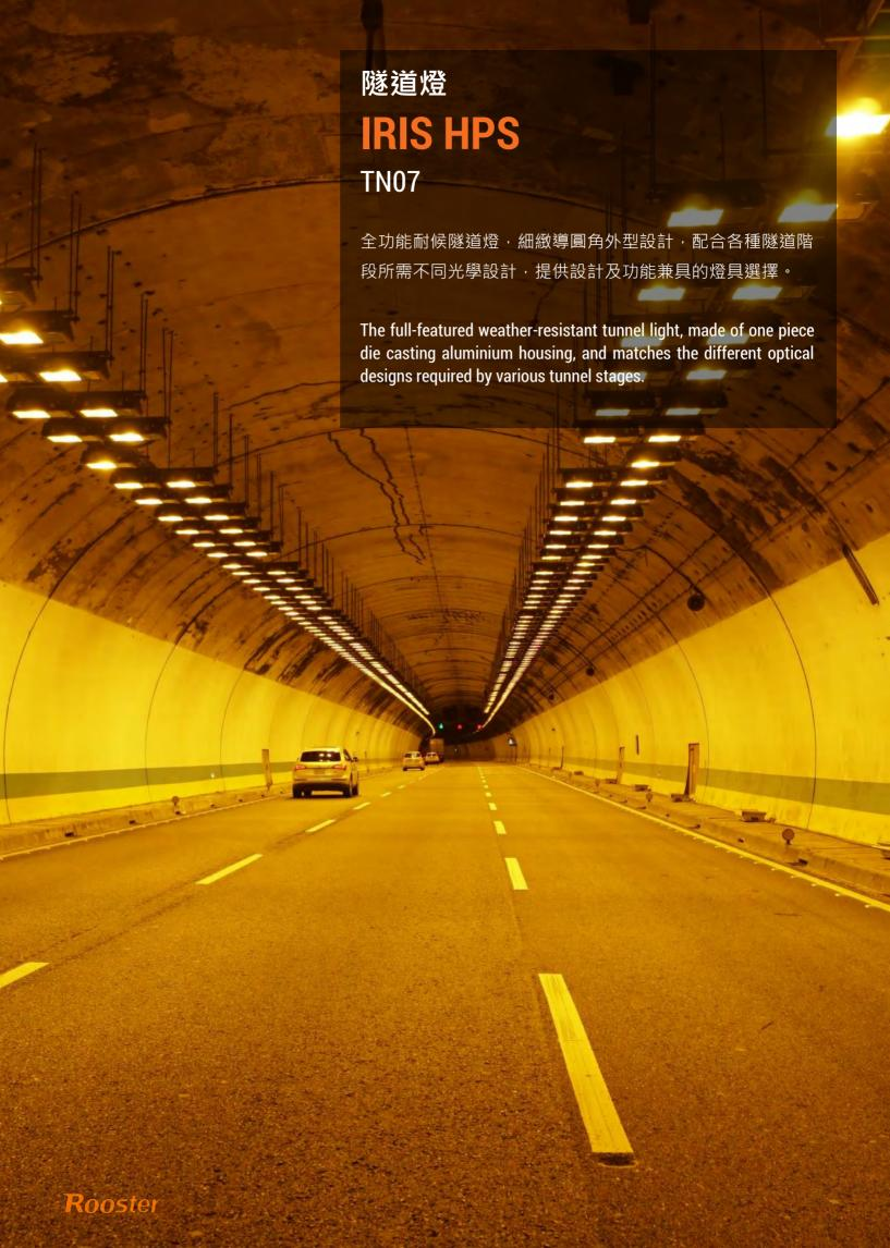
外罩 | 壓鑄鋁Cover | Die casting aluminium面框 | 壓鑄鋁Frame | Die casting aluminium燈罩 | 強化玻璃Lamp cover | Tempered glass
